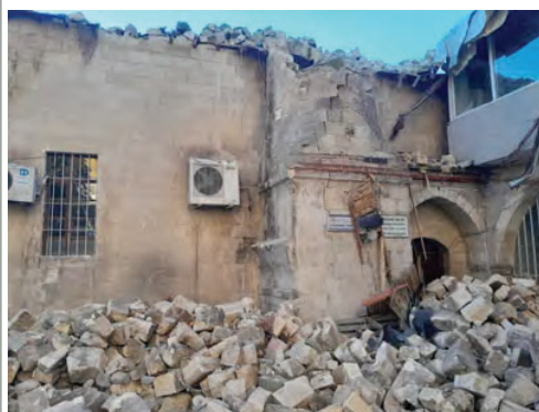
Out-of-plane mechanism observed in Adiyaman Kab Mosque on 17 February 2023 (Emre Kishali archive).
