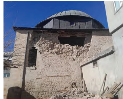
The collapse of the masonry walls and roof observed in Adiyaman Ulu Mosque on 17 February 2023 (Emre Kishali archive).
