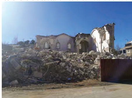
The collapse of the masonry walls and roof observed in Adiyaman Ulu Mosque on 17 February 2023 (Emre Kishali archive).
